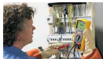
Insulation test at a distribution panel
